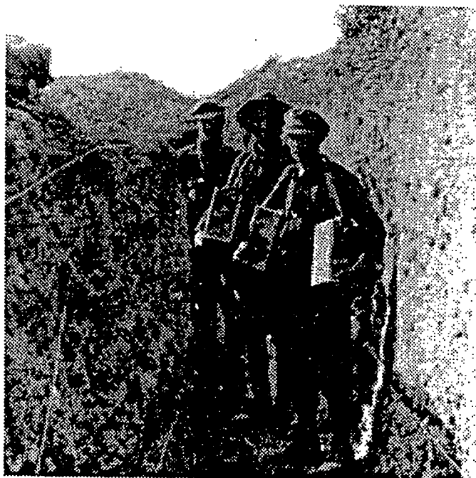
Figure 3. Carrying water in the trenches.
